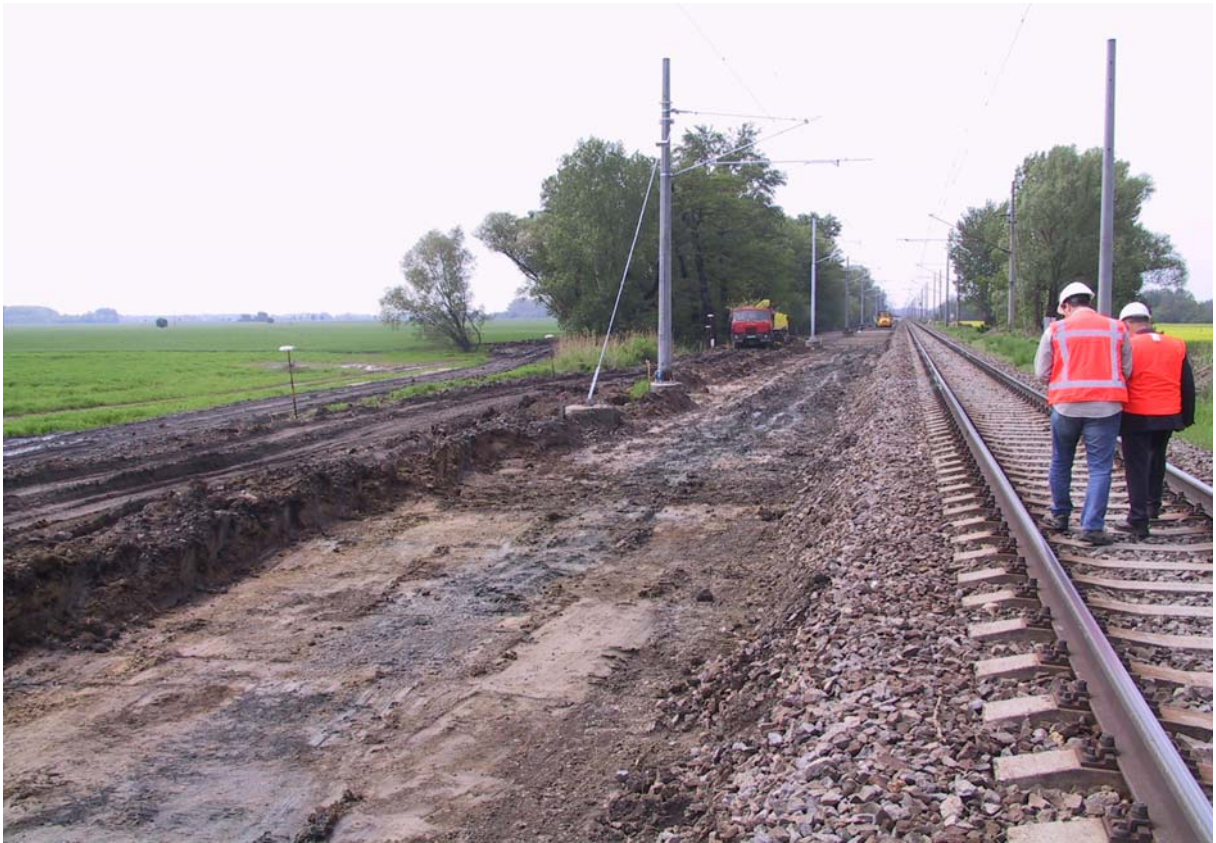
Fig. 4 Brestovany – Leopoldov, track number one, earth subgrade before reconstruction
