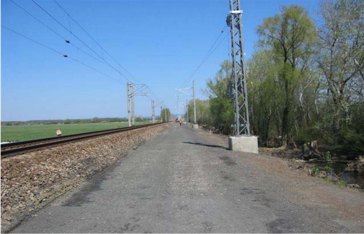
Fig. 6 Brestovany – Leopoldov, track number one, modified and compacted earth subgrade
