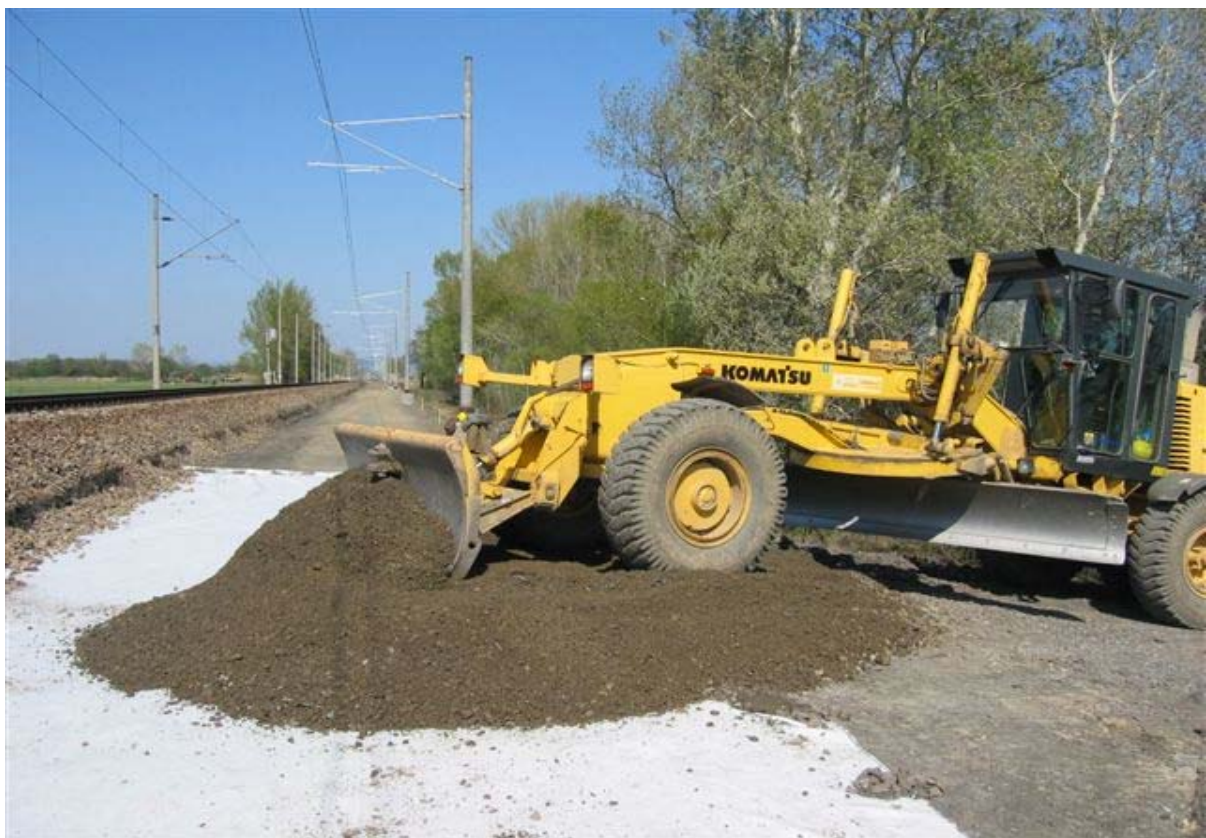
Fig. 9 Brestovany – Leopoldov, spreading the base layer of crushed gravel fraction 0 – 32 mm
