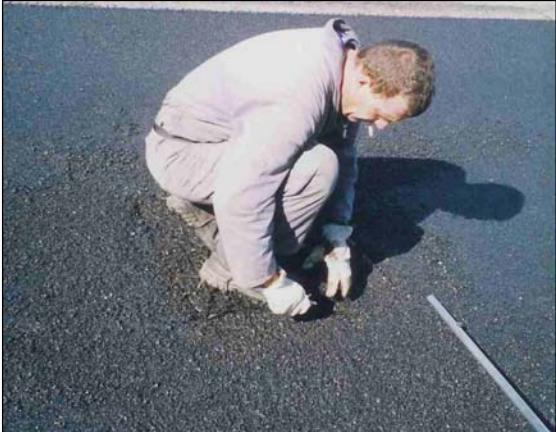
Fig. 10 – Manual cut of the Geogrid around hitches and traps
