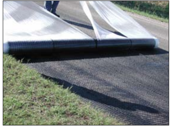
Fig. 3 – The ARTER® GTS A geogrids are rolled with a very thin polyethylene sheet
