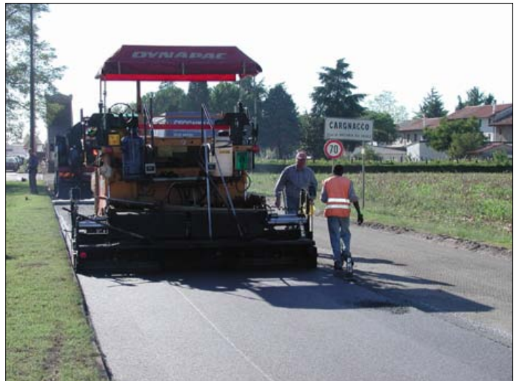
Fig. 15 - Asphalt surface results smooth and uniform
