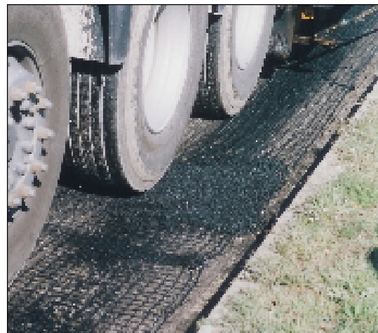
Fig.9 – A small quantity of asphalt on the first metre of Geogrid and along side edges allows to keep the roll in the right position.
