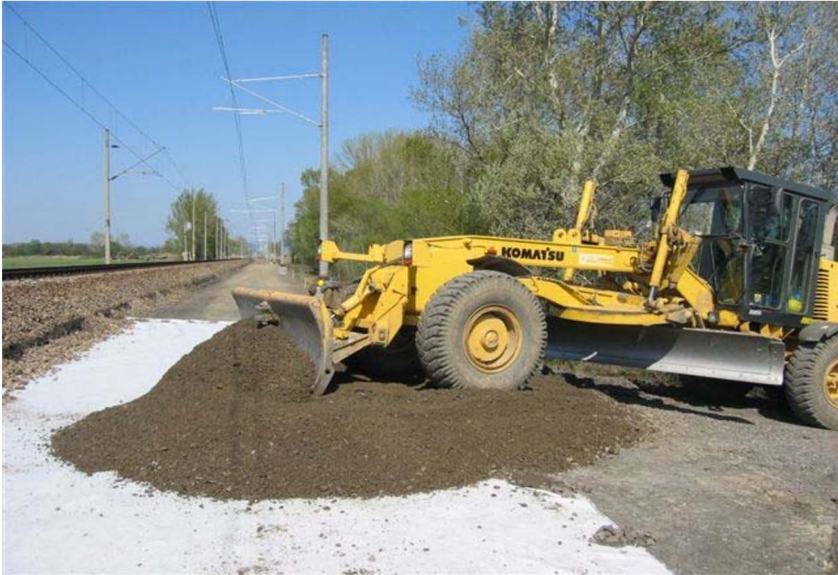
Brestovany – Leopoldov, spreading the base layer of crushed gravel fraction 0 – 32 mm
