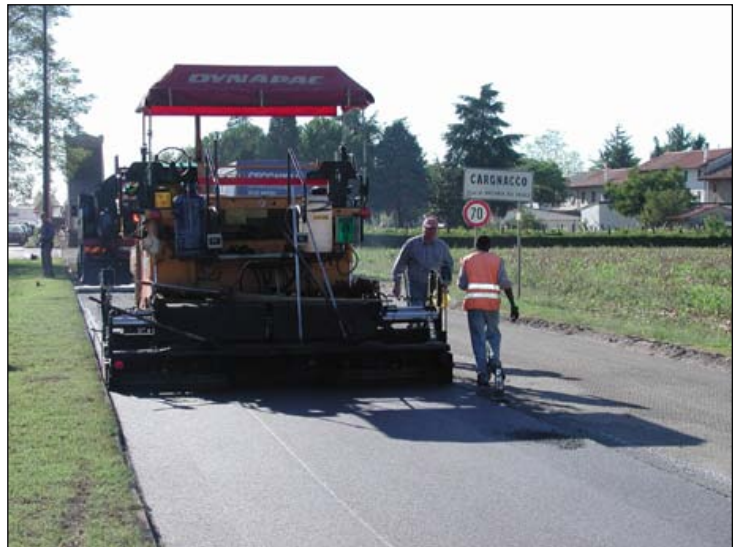
Fig. 15 - Asphalt surface results smooth and uniform
