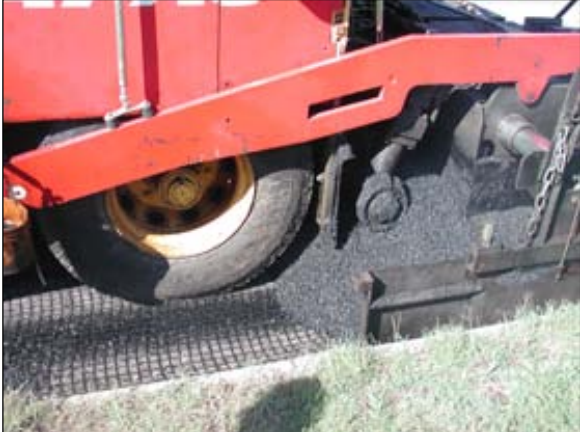
Fig. 11 – Laying the asphalt in 60 mm loose thickness by a finisher
